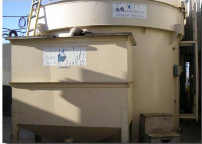
Pollutants literally float to the top in the Dissolved Air Floatation (DAF) Tank
