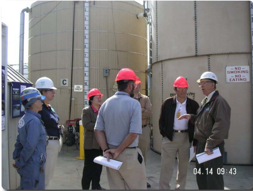
(Left) Myrna Contreras & Sara Giobbi (NASSCO), Tam Doduc & Jerry Secundy (State Water Board), Steve Clarey (NASSCO) tour NASSCO's Wastewater Treatment Facility.
