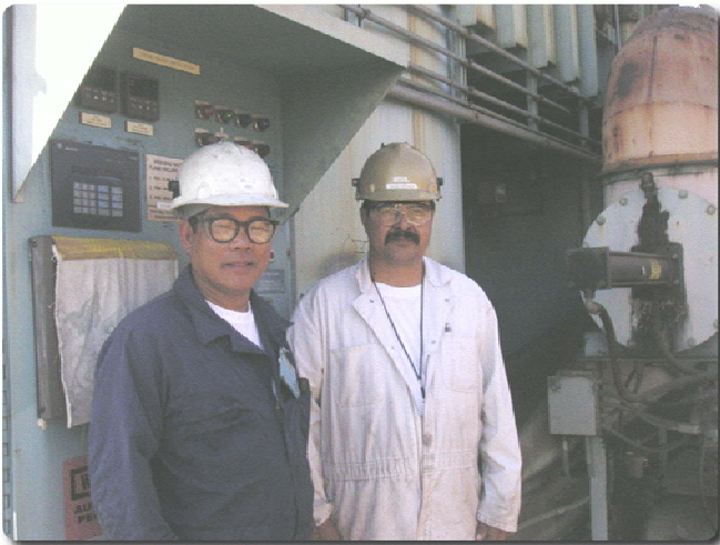
Valentino Ibay, Maintenance Electrician, and Sergio Ascencio, Wheelabrator Foreman, at the Primeline #1 Thermal Oxidizer.
