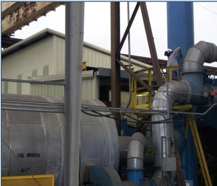
APCD Inspector Ian Morris sets up NASSCO's Prime Line #2 Oxidizer for a source test.
